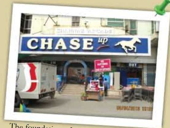
The foundation of the fourth departmental store was laid in July 2010 at Shaheed-e-Millat Road (Bahadurabad).
